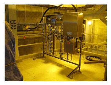
Figure 1: Celgar's FITNIR Analyzer Sampling Skid: six sample streams (RGL, CGL, WW, WL,#1C, #4C), shown without roof and plastic cover.
